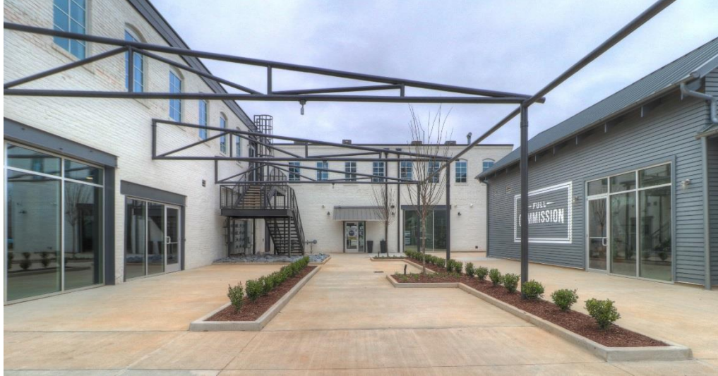
Woodward & Park space at Larkin on Memorial appears to the left with ample patio space out front. Photo credit: Stephen Rickard
